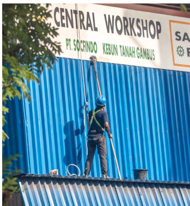
📷 Providing safety equipment is a responsibility we take seriously
