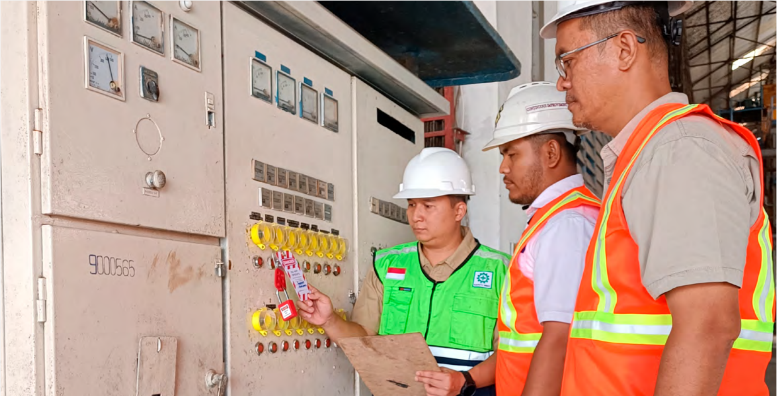
📷 OSH officer conducting training on the implementation of the LOTO (Lockout/Tagout) system at the mill
